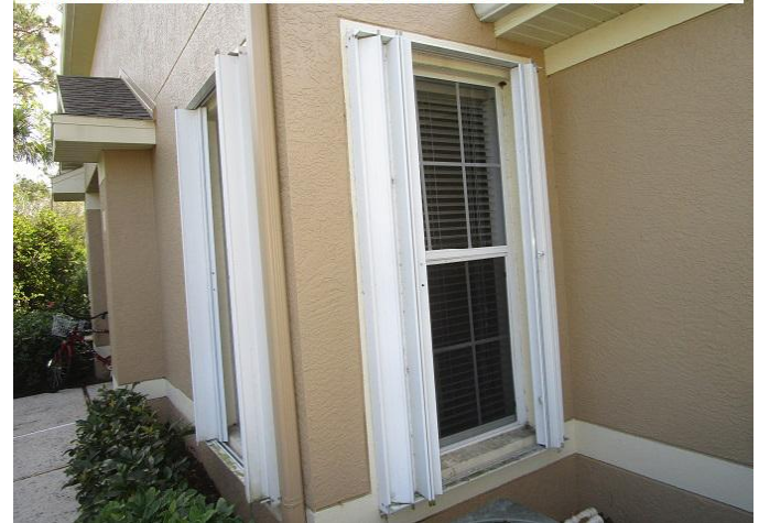
#7) opening protection: original non impact windows- some w/shutters
