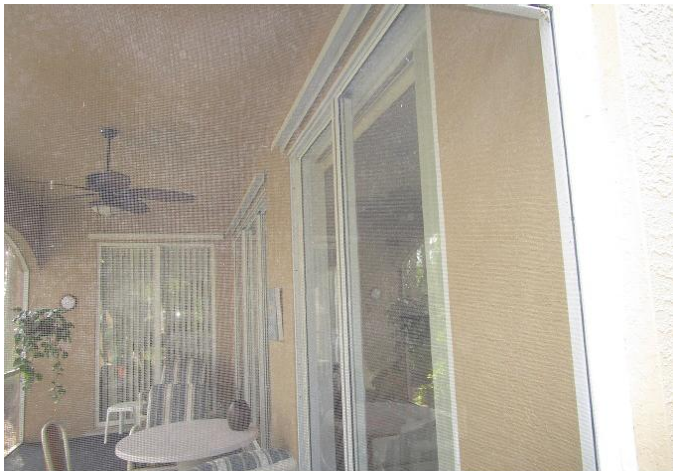
#7) opening protection: non impact sliders- some w/shutters
