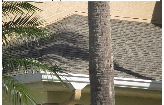
#2) roof covering: 2016 dimensional asphalt shingle HIP style roof #16355-0 issued 2/23/2016
