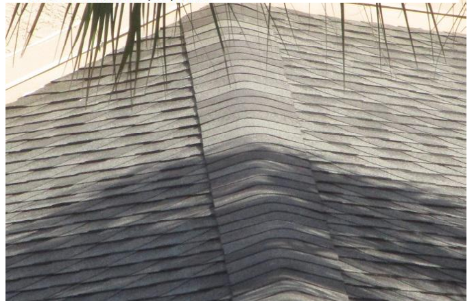
#2) roof covering: 2016 dimensional asphalt shingle HIP style roof #16357-0 issued 2/23/2016
