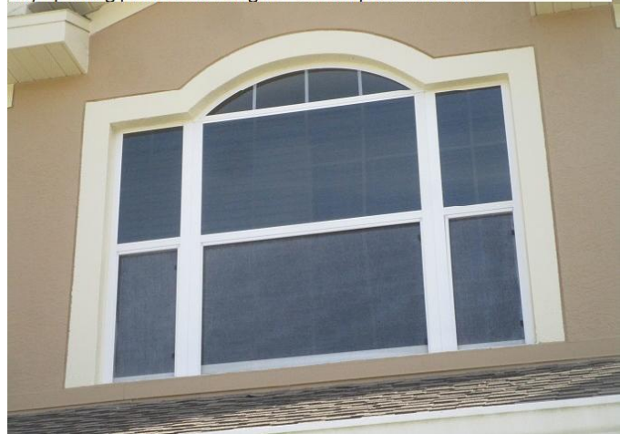
#7) opening protection: original non impact windows
