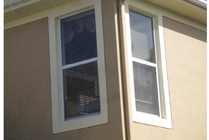
#7) opening protection: original non impact windows
