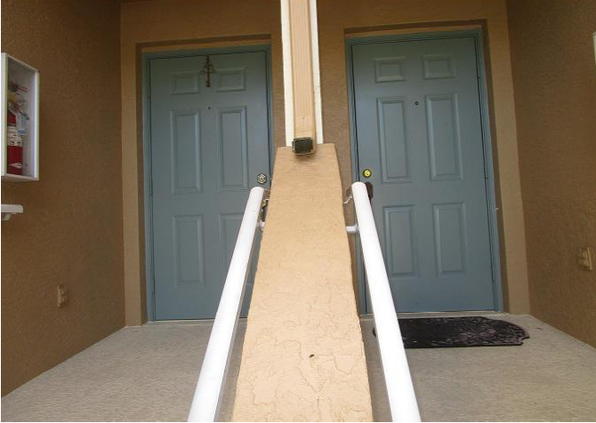
#7) opening protection: metal clad door
