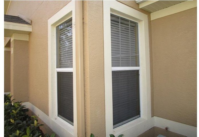
#7) opening protection: original non impact windows
