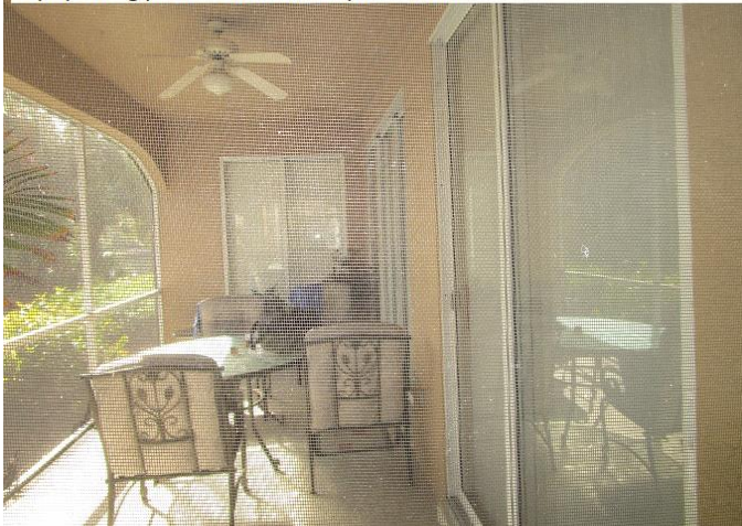
#7) opening protection: non impact sliders
