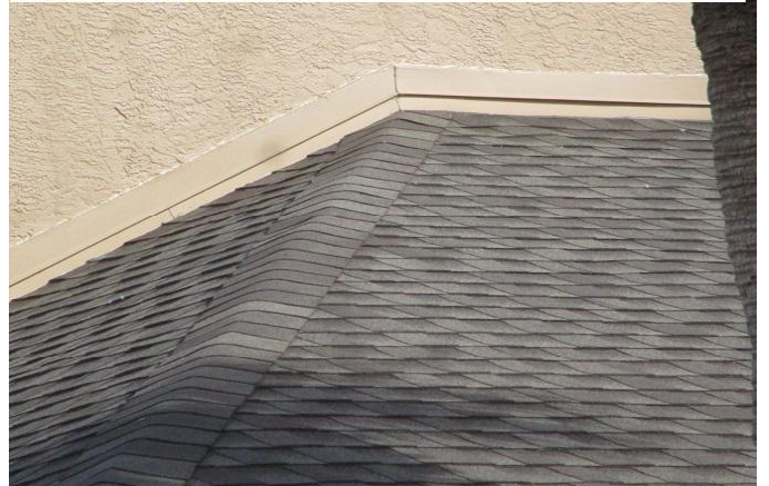
#2) roof covering: 2016 dimensional asphalt shingle HIP style roof #16359-0 issued 2/23/2016
