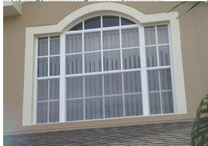
#7) opening protection: original non impact windows
