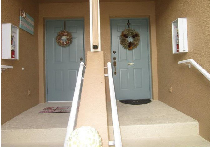
#7) opening protection: metal clad door
