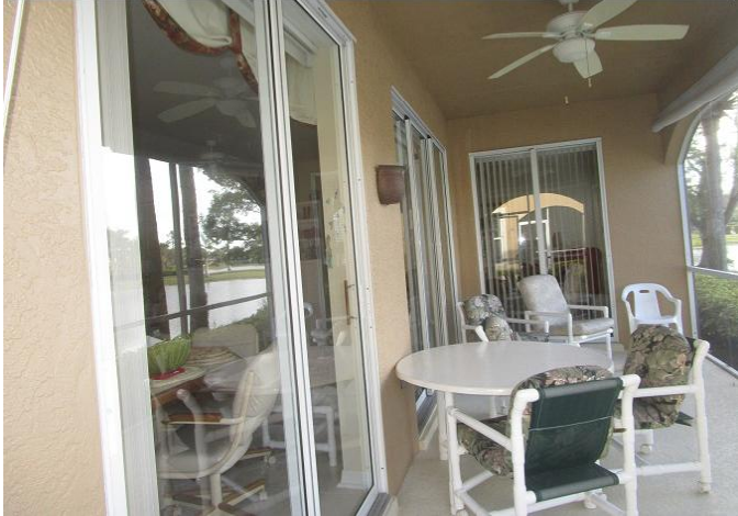
#7) opening protection: non impact sliders
