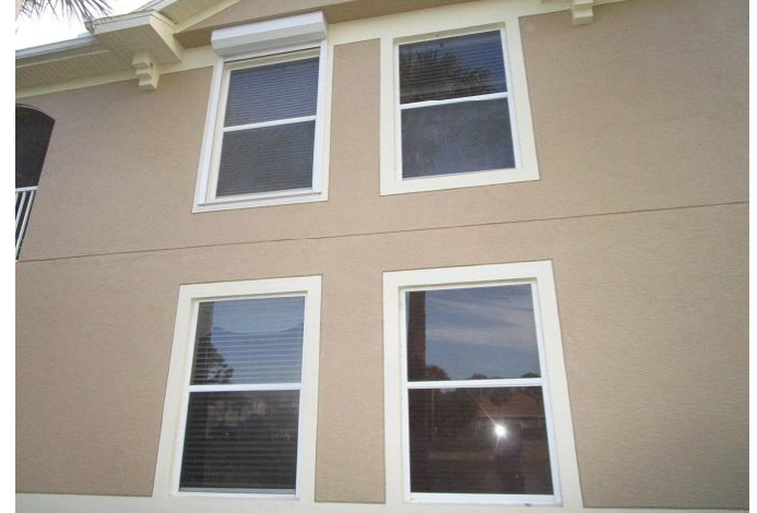
#7) opening protection: original non impact windows- some w/shutters
