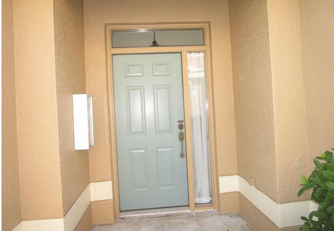
#7) opening protection: metal clad door w/non impact transom & sidelite
