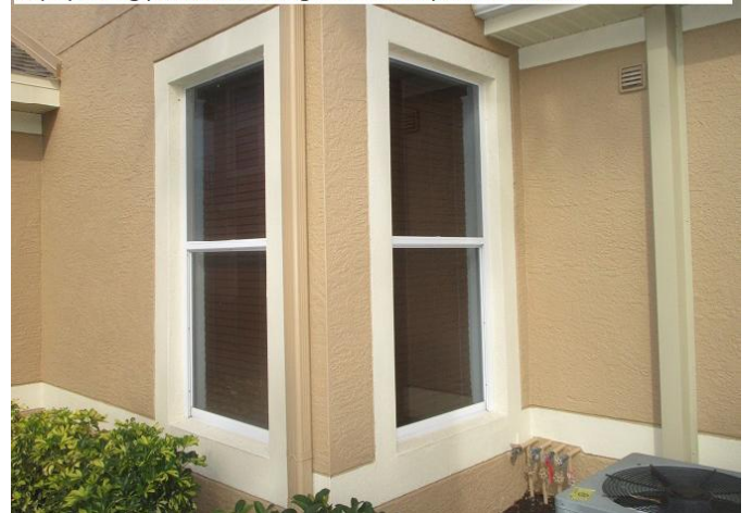
#7) opening protection: original non impact windows
