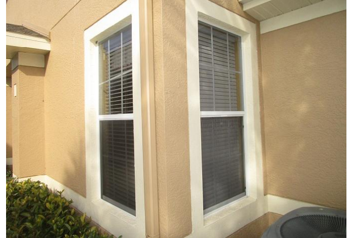
#7) opening protection: original non impact windows
