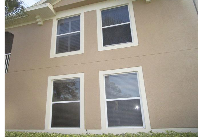
#7) opening protection: original non impact windows
