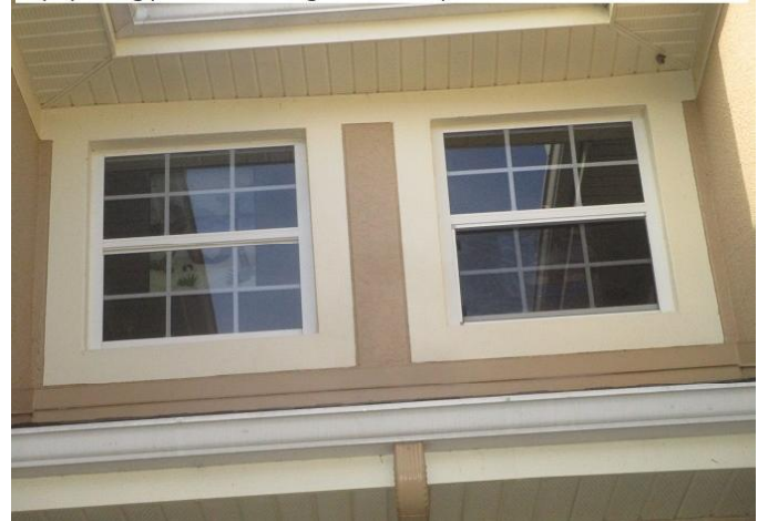
#7) opening protection: original non impact windows
