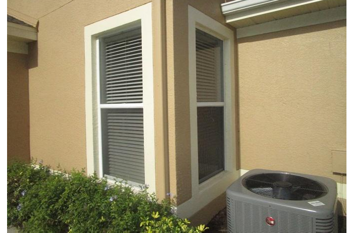
#7) opening protection: original non impact windows
