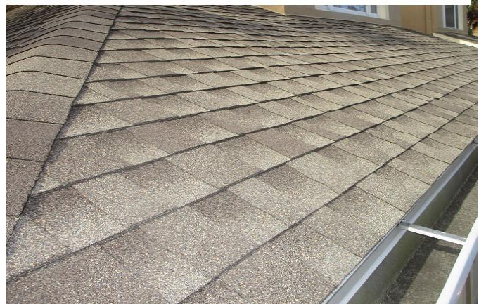
#2) roof covering: 2016 dimensional asphalt shingle HIP style roof #16264-0 issued 2/12/2016
